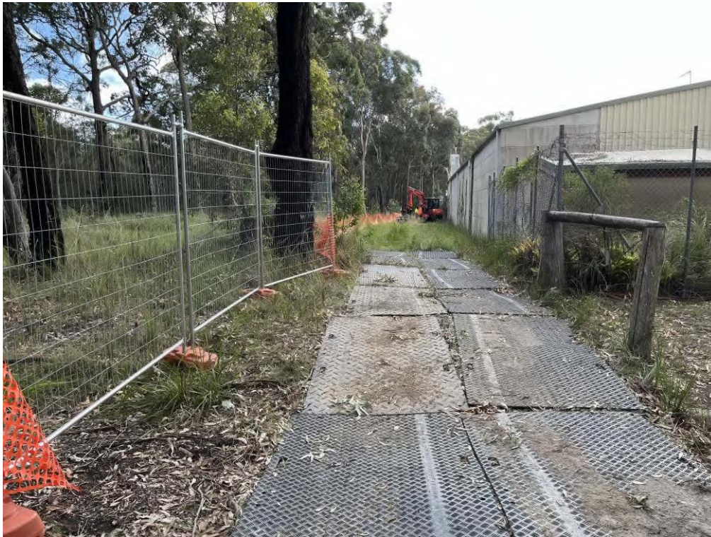
Figure 2: Fencing protecting trees and other habitat features outside of the EW1 clearing footprint
